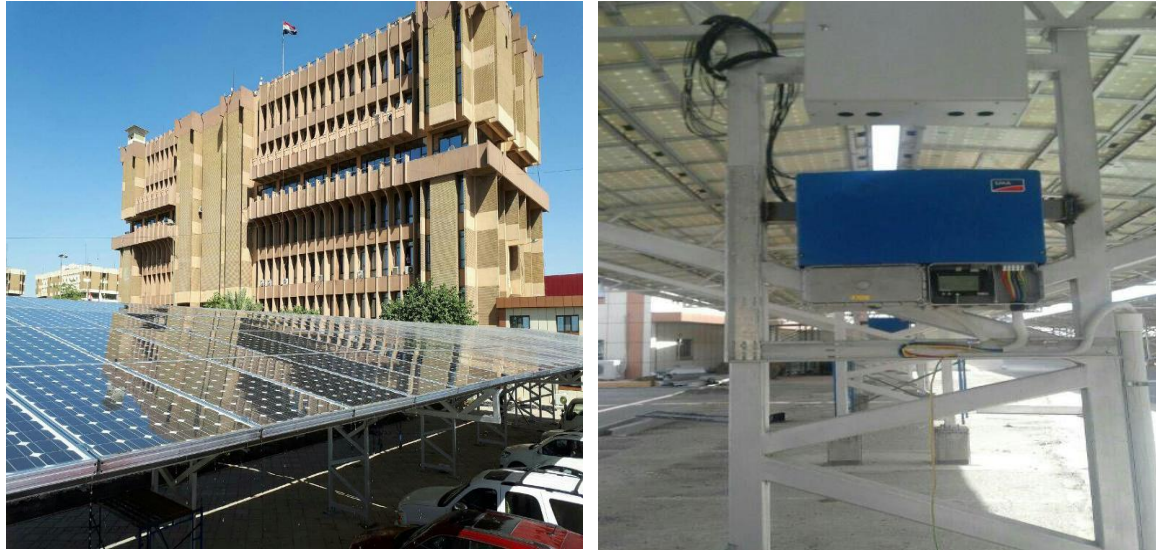
Figure 4. This figure shows the real PV system grid tied that has been installed at Baghdad Site, (a) Solar Array (Sharp 175Wp); (b) Solar Inverter (SMA 25kW).
